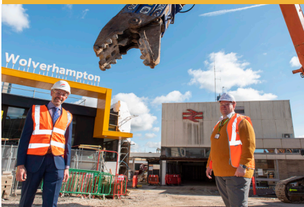
Cllr Stephen Simkins (CWC) and Malcolm Holmes (TfWM Director of Rail) marking the start of Phase 2 demolition (old station building)
